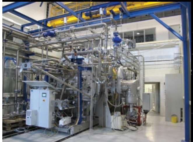
Vacuum system for E-beam high heat thermal loading
